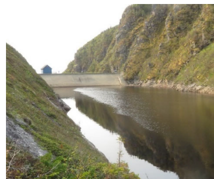
Rose Blanche hydroelectric plant forebay dam.
