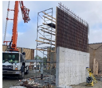
Civil work ongoing at Memorial Substation in St. John's.
