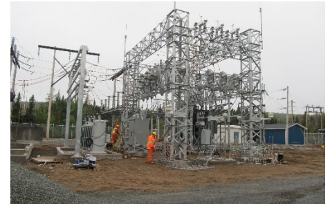
Construction at Gambo Substation in Central Newfoundland.
