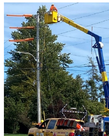
Construction on WAV-01 distribution reliability initiative project near Chapel Arm.
